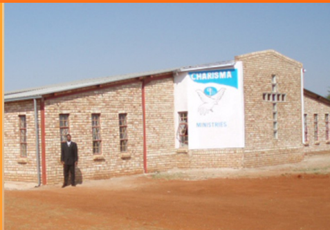
CHURCH BUILDING : Assisted with building more than 83 churches.
